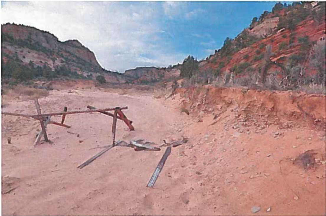
Knocked down fence along route 20WSA.
