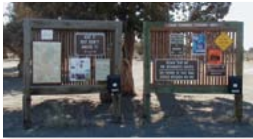
The vertical see-through slats are a nice design, but not functional. Wind and rain blowing through the slats rips and saturates posters.
