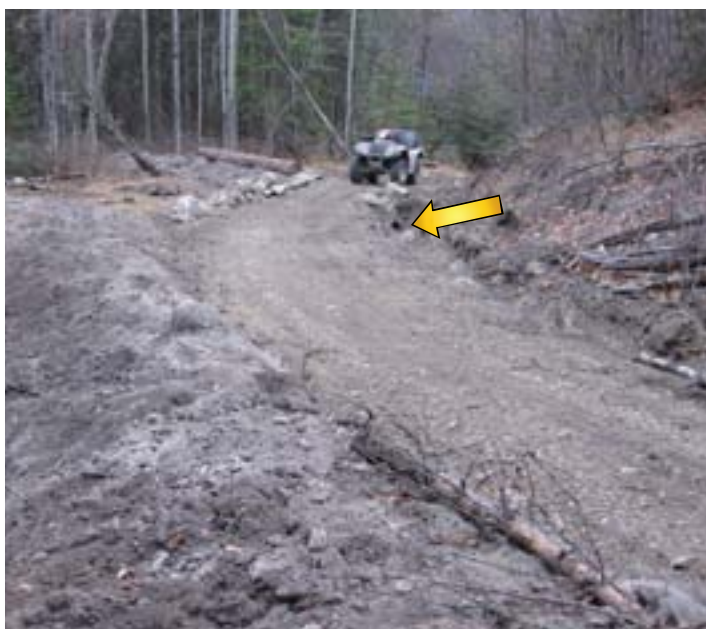
This trail runs up a draw which has springs on both sides of the trail. In the wet season, this flat area at the outlet of the draw would become a saturated mudhole. Ditches were cut down both sides of the trail to intercept the spring water and drain the trail tread. The excavated material was used to raise the trail elevation and a culvert was installed to drain the ditch water under the trail (arrow).
