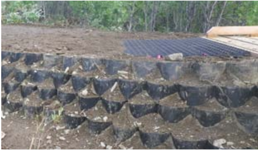
The fill for this bridge approach and bridge abutments has been constructed in layers of geocell with a good soil and rock mix. Note the grass paver panels to insure a smooth transition onto the bridge deck.
