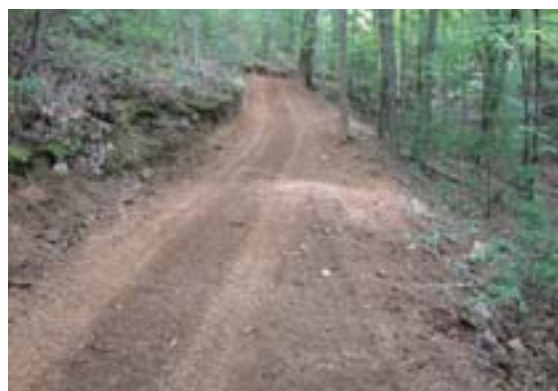
The same site after the solution was implemented: an improvement for the riders, the resources, and a sign of professional management.
