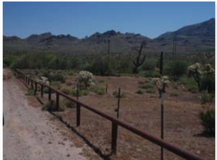
With no other materials readily available and in an area prone to vandalism, these pipe barriers are a good choice.
