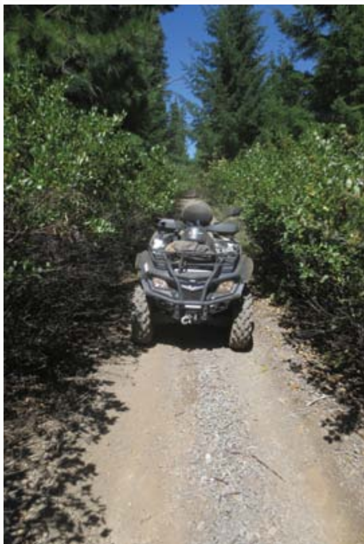
Nothing was done to this road except remove the full-size vehicle use and stop vegetative maintenance. In this good growing environment, it has quickly converted to trail width complete with leg slappers. It would have been better to have a serpentine alignment, but at least in this segment, the road corridor is obscured.
