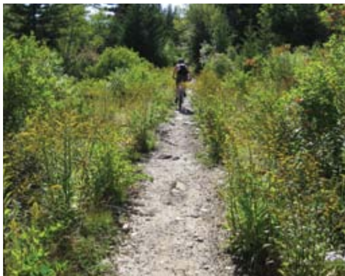
As with many structures, there are short-term impacts upon implementation. Don't let those impacts deter your design decision. Above, a section of recently constructed turnpike on a road-to-trail conversion. Right, the same section one and a half years later. High, dry, and a great single-track experience.
