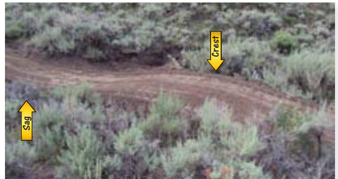
This is a nicely constructed rolling dip. Notice the distance from the sag to the crest and notice how the grade smoothly rolls into and out of the dip.
