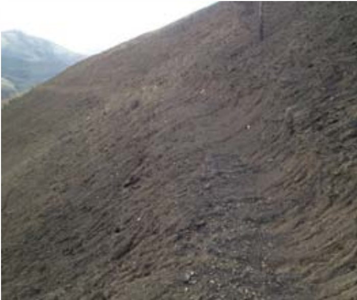
A high-intensity rain storm shortly after this fire resulted in a massive overland flow that washed across this trail, filling it with mud.
