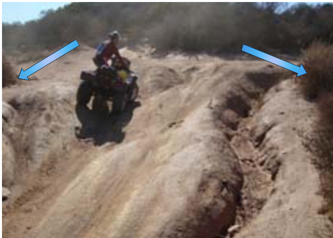
Ruts contribute to challenge and so does this clay soil. To stabilize this, explore options to drain the water off before it gets to this slope (arrows).
