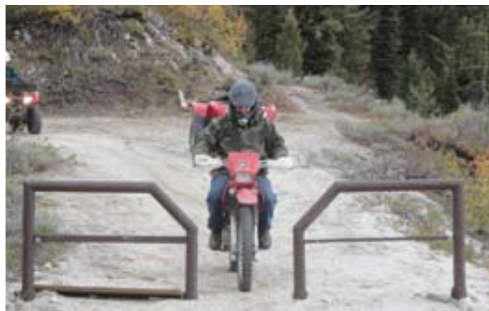
Steel pipe is vandal-resistant and sends a stronger message when one is needed.
