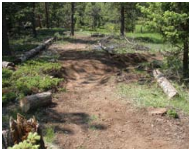
A nice lead-off ditch was constructed to drain a rolling dip, but as riders' eyes scan this area, it is difficult to determine a ditch or a trail going off to the right. A millisecond of uncertainty can draw a rider into the ditch. To avoid this, it is a good practice to place a small log across the ditch entrance so it spans the ditch without blocking the flow of water.
