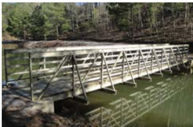
With transport and assembly advantages, a fiberglass pony truss bridge can work well in a variety of settings.
