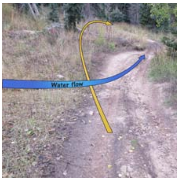
When constructed, this trail was outsloped so the small drainage entering from the left would drain across the trail. Through compaction, displacement, and lack of maintenance, the trail bed is now lower than the ground on the downhill side, so the water runs down the trail. Now, a rolling dip should be installed here. In reality, there was an error in the initial location and the alignment should have pitched up on the arrow line to create a grade reversal and positive drainage.
