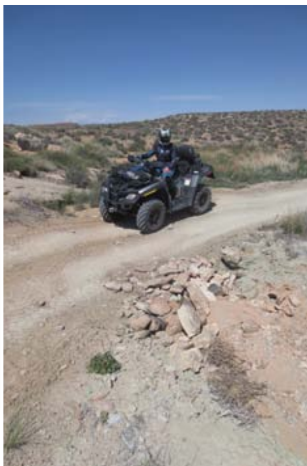
This trail has been outsloped to provide drainage. The rocks at the outlet serve as energy dissipaters and are a nice touch.
