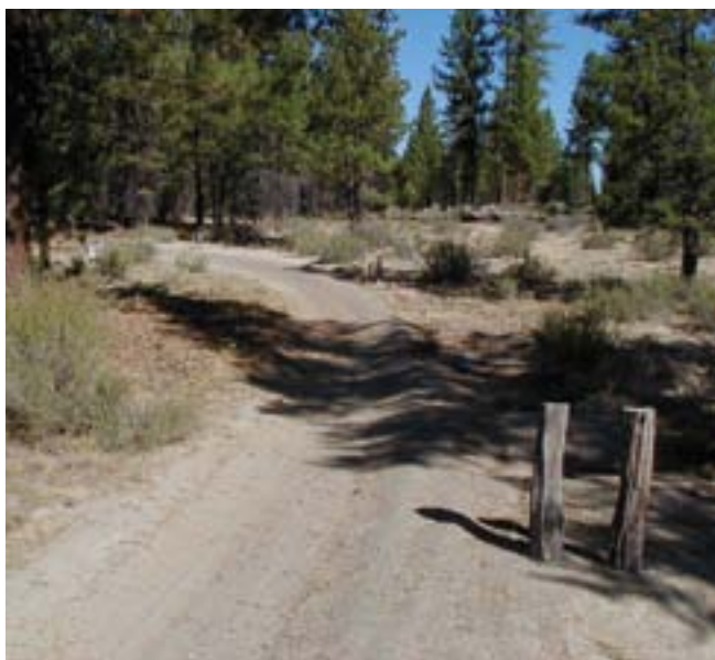
This road to trail conversion is adjacent to a major trailhead and campground and the kiddies kept riding the ripped up portion. We finally installed these juniper posts to deter that activity and they worked. Utilize the 4E's to implement, evaluate, and adjust as necessary.
