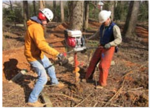
Gas powered augers save time and hands for sign post or fence installation.
