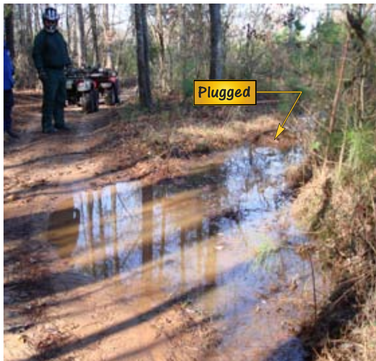
Avoid flat ground. Even with outslope, the water won't drain off the trail if it has no place to go. This lead-off ditch has plugged up or was under-sized and needs maintenance. A drainage sump may be a better alternative.
