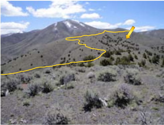
This trail would have had less visual intrusion on the landscape if it had been located in the trees (arrow), but the terrain was steeper on that slope and it lacked places for enough climbing turns to gain the elevation that this trail needed to gain to hit control points.
