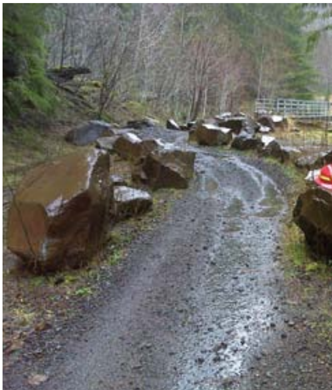
Rocks define a serpentine corridor which slows the riders before approaching the bridge. In this wet environment, this old road corridor will quickly transform into a great trail.
