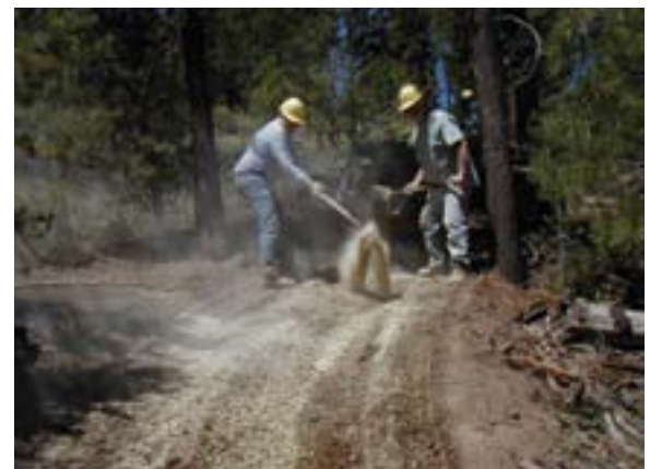
When the spreader box plugged up, the eyeball measuring and hand distribution methods were used.
