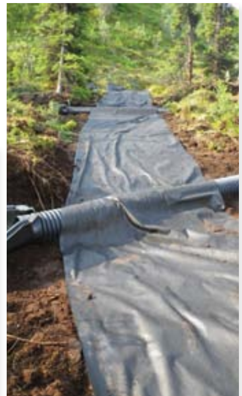
Geotextile is being put down to provide separation and reinforcement on this Alaska trail.
