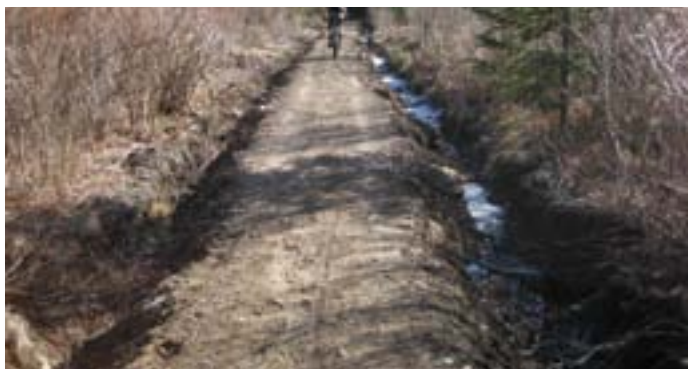
As with many structures, there are short-term impacts upon implementation. Don't let those impacts deter your design decision. Above, a section of recently constructed turnpike on a road-to-trail conversion. Right, the same section one and a half years later. High, dry, and a great single-track experience.
