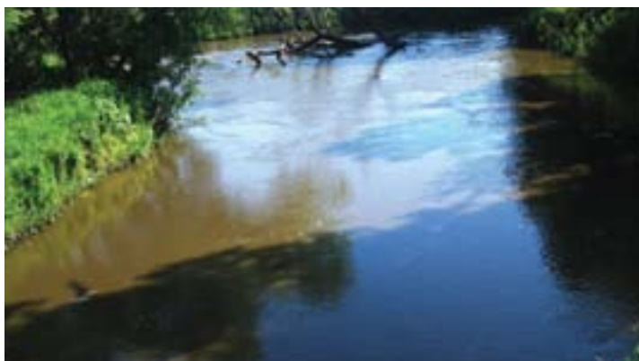
After searching ¼-mile upstream & downstream, this was the only bridge site that would work to cross this very sensitive stream. It was not perfect (few are), but there was topographic relief on both sides, a straight channel, and minimal scour of the banks. This site became a positive control point. The next challenge was to get the trail down to it.
