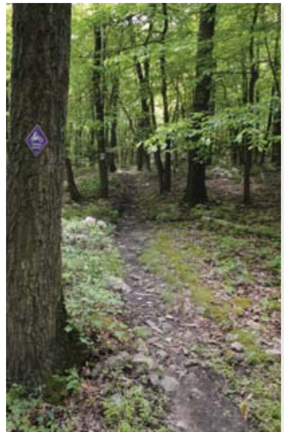
This heavy tree canopy helps protect this trail from splash erosion. The high rock content in the tread will add to the durability of this trail.
