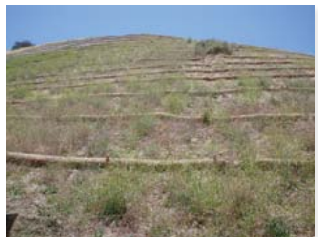
Above, rows of wattles staked closely together as part of the rehabilitation of this steep slope.
