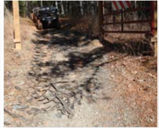
The fill layer over this installation was not maintained. Direct tire impact displaced the material in the cells and destroyed the integrity of the structure.
