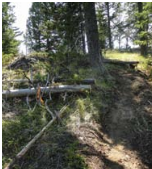
The trail was designed (flagline) to go up a rock step-up which would have been consistent with other features on this trail, but the builder chose to avoid it by moving off to the right and putting in a 90 degree turn above the tree. The result is a loss of a challenge feature, tread durability, and flow.
