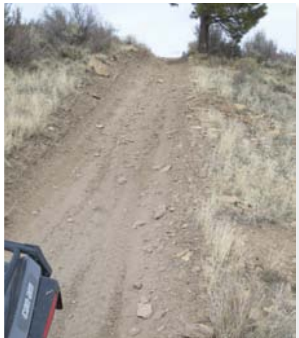
The high rock content on this grade has made it durable. The grade is steep (25%) but short (50'). In spite of a dramatic increase in use, this slope has changed little in 15 years of monitoring.
