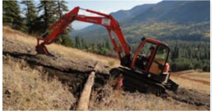
This excavator is rehabbing old hillclimb trails. It is scarifying the trail, installing waterbars in a herringbone pattern, and strategically placing logs that divert water and deter riders.
