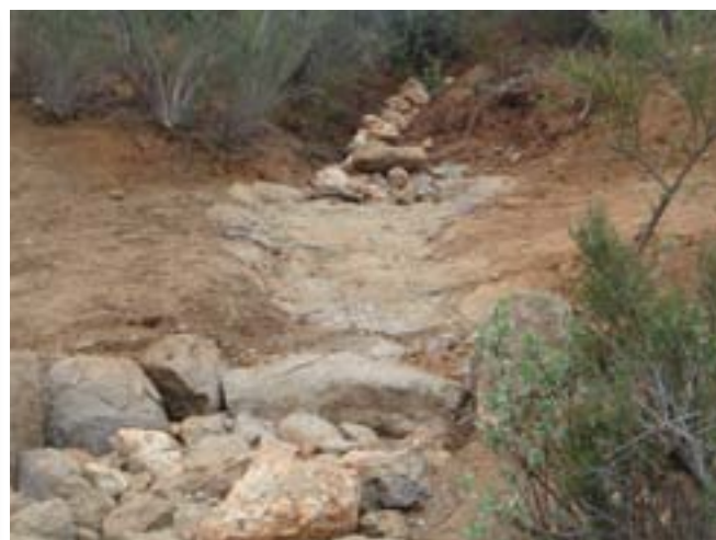
This seasonally wet crossing has been hardened with cobble-sized rock. This is simple and effective and there is no culvert to clean out or plug up. In arid country, runoff from a high-intensity thunderstorm can wash out a culvert, but a hardened drain will likely endure.
