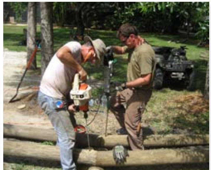
Drills and bits are invaluable for on-site structure assembly.
