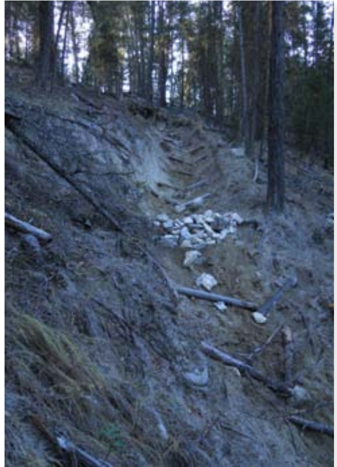
Here, water quality and sedimentation were an issue. Woody debris was placed in a herringbone pattern between rock check dams in a heavily eroded trail leading to a creek that feeds the community water intake.
