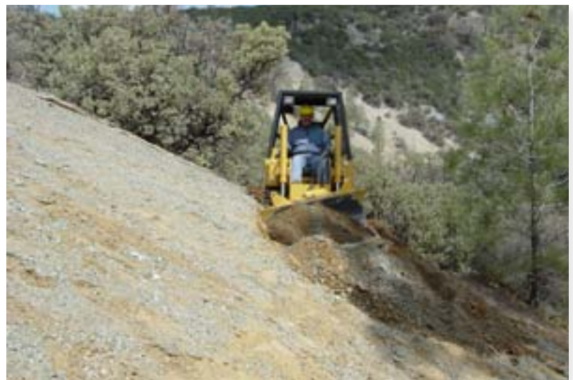
A 6-way blade makes short work of trails on steeper ground.
