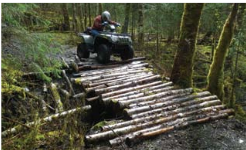
In the backcountry, corduroy is sometimes used as a bridge. This is not a recommended practice and should be considered a temporary bandage due to its structural instability. Grade should be avoided with corduroy, especially in wet climates. The slippery, uneven logs on this installation make it a liability.
