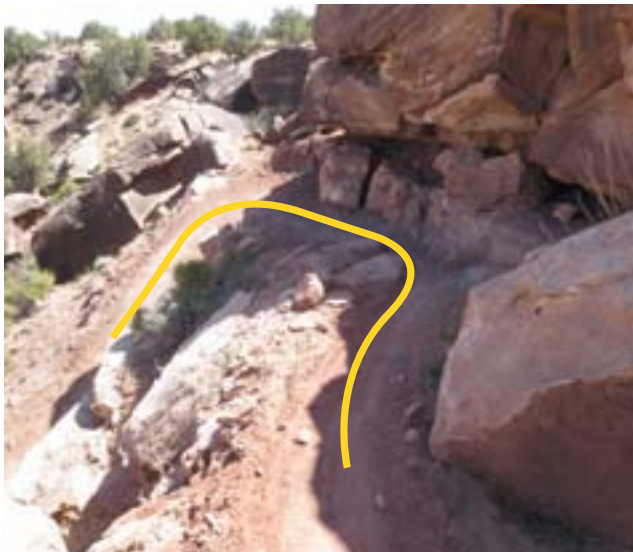
This switchback has almost no landing, no flattened approaches and is not easy to ride because it consists of two 90 degree turns rather than one circular curve. Obviously, the geography here limited options and that's the real world. This is also a most difficult trail, so the switchback is consistent with the TMO.
