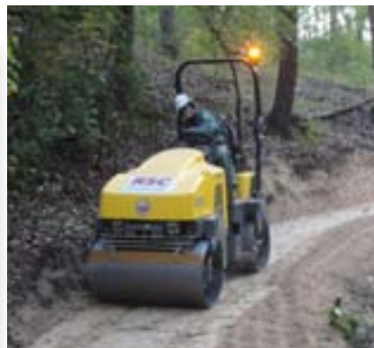
Moist soil will compact better than dry soil, so try to time compaction operations during periods of favorable moisture content.
