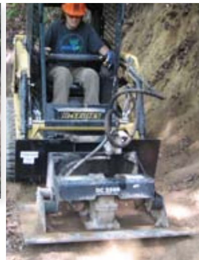
These handy vibratory plates will not exert the same compactive effort as a smooth drum roller, but they do a good job smoothing and compacting the surface of the tread. One advantage of compaction attachments is that they can be raised by the equipment to avoid root or rock sections.
