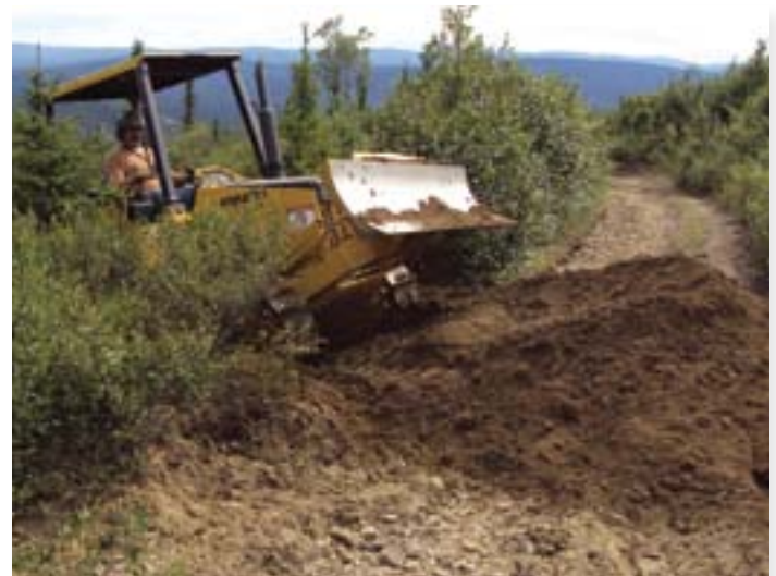
The best way to start building a rolling dip is to borrow as much material for the crest as possible by using lead-off ditch or drainage sump excavation. Excavating the sag to build up the crest increases the grade going into the dip, reduces the flow of the dip, and can make it more difficult to drain water out of the dip.
