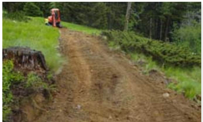
Equipped with a 6-way blade, this excavator is a versatile trail making machine.
