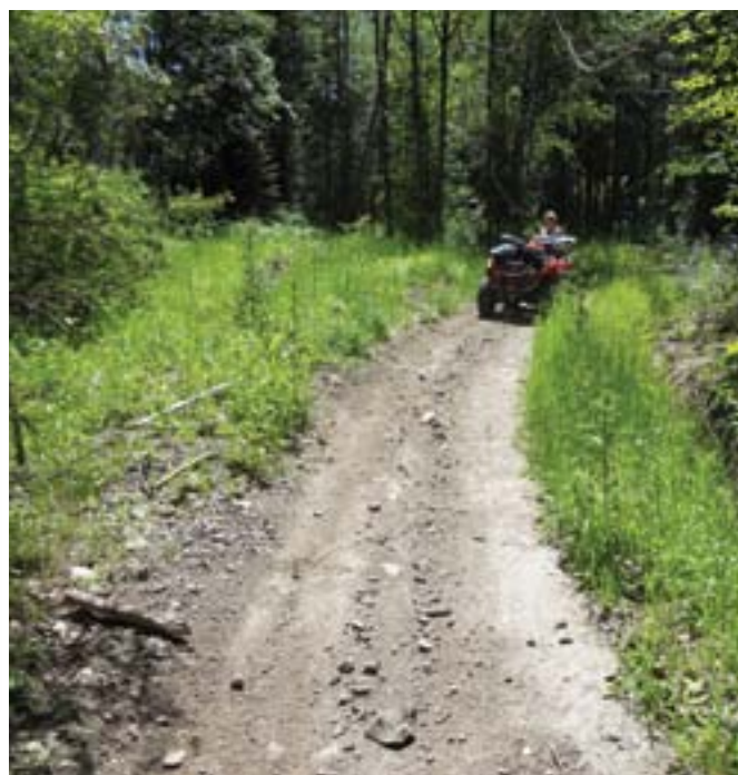
Three years later, the trail tread is high and dry and lush vegetation is growing in the ditches. Use the 4Es. Evaluation is a valuable tool to show what is working (or what isn't). Pictures like these can give managers positive encouragement, can mollify critics, and build support with stakeholders.
