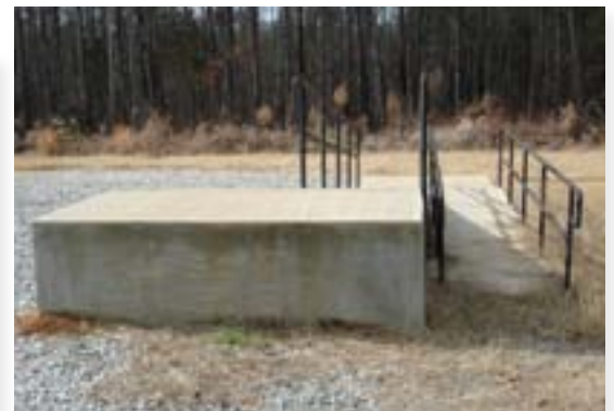
With the concrete and the railing, this ramp was expensive to construct. It is accessible, but the approaches in the gravel probably aren't. If the concrete truck is going to be there, why not pour a concrete parking pad and approach to the ramp?
