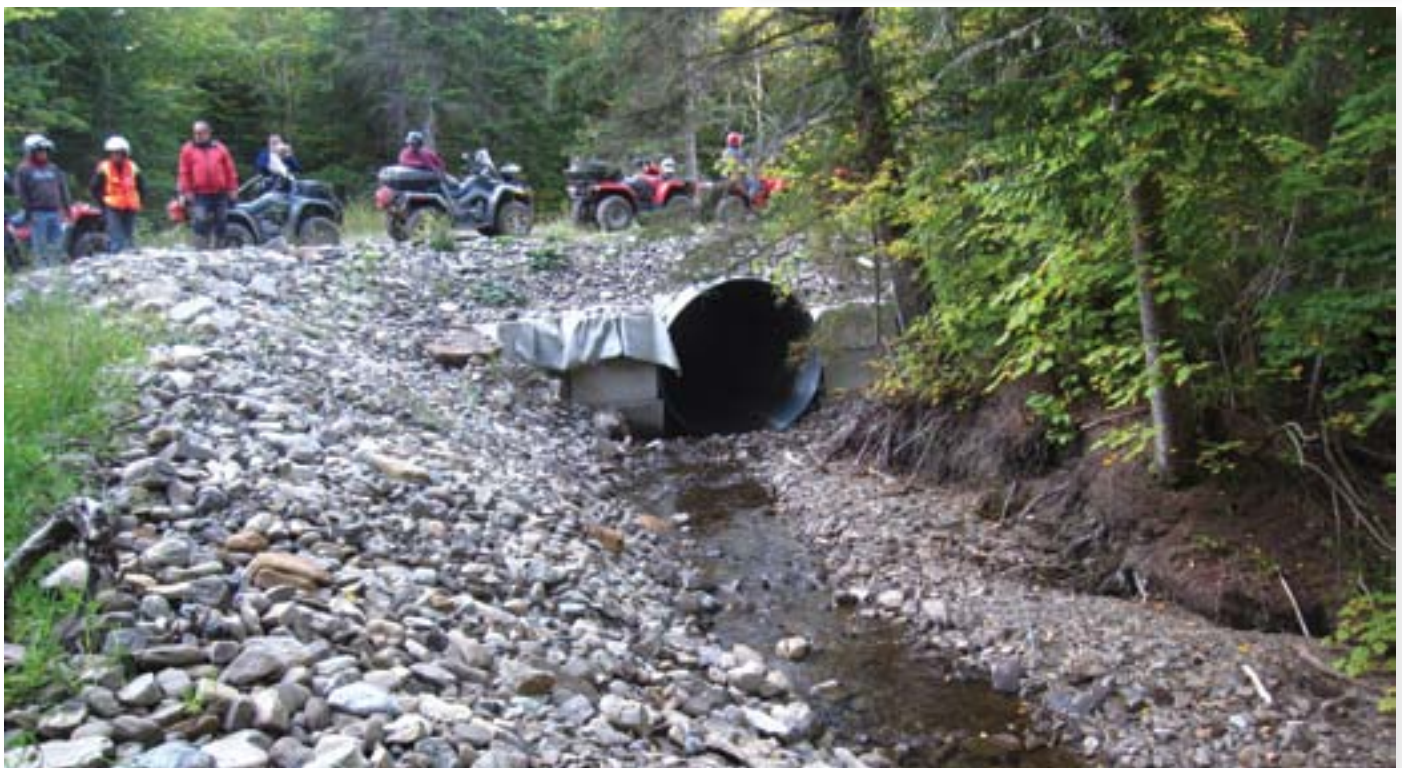
Here, water quality and sedimentation were an issue. Woody debris was placed in a herringbone pattern between rock check dams in a heavily eroded trail leading to a creek that feeds the community water intake.
