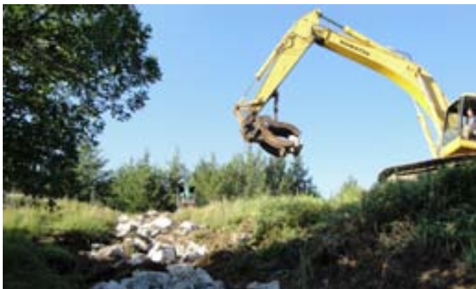
Need more reach? Not a problem as this excavator places a blanket of energy dissipaters in this drainage.
