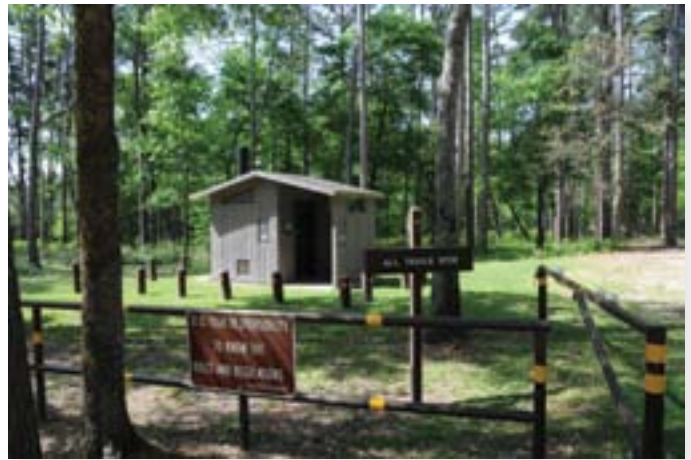
Neat, clean, and functional, this trailhead provides good customer service and communication.
