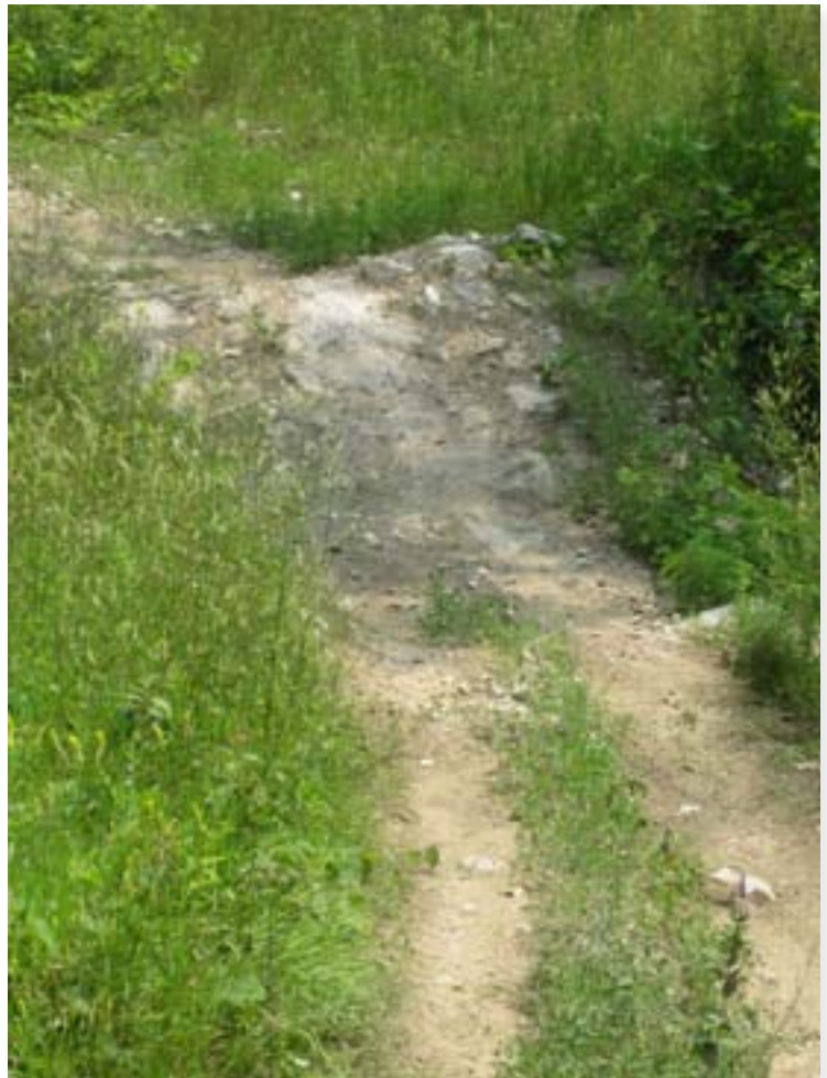
This rock outcropping was used as a pivot point for a curve in the trail. The rocks help stabilize the soil and increase the variety in the trail.
