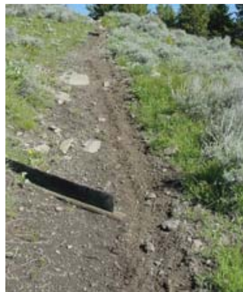
This trail has a long, steep grade, and poor soil type; all ingredients of non-sustainability. Like the rolling dips in roads, these belted waterbars reduce the distance that water runs thereby reducing the size of the tread watersheds. Unfortunately, these won't work. As you can see, riders are already starting to ride around the waterbars and as soon as this happens, ruts will form to channel the water and bypass the waterbars. The result is failure. A bandage fix like this is all too common and it doesn't address the root of the problem: poor trail location.
